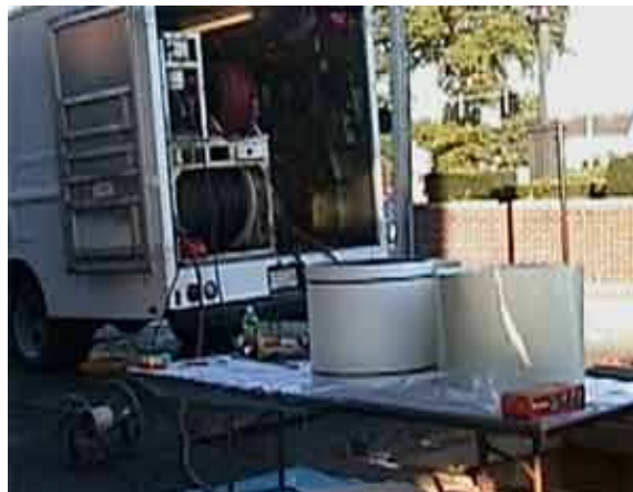
Gas Sealer™ Sleeves ready for installation
